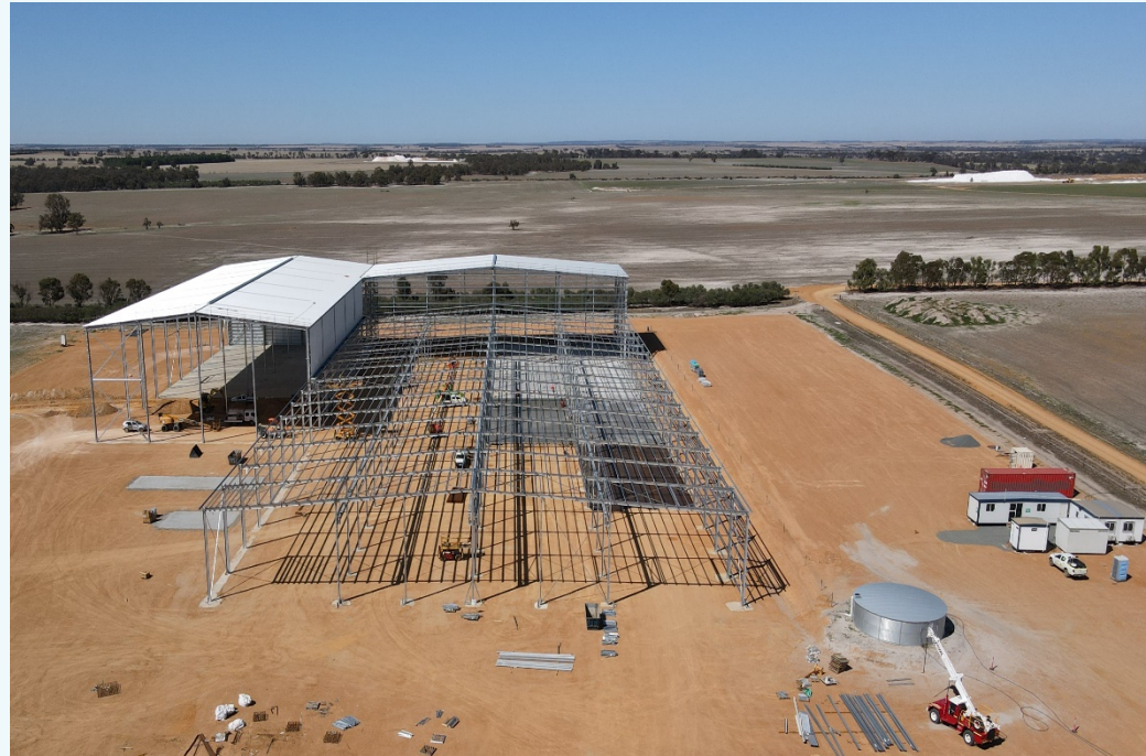
Ongoing plant construction at Wickepin, open pit operations in the background
